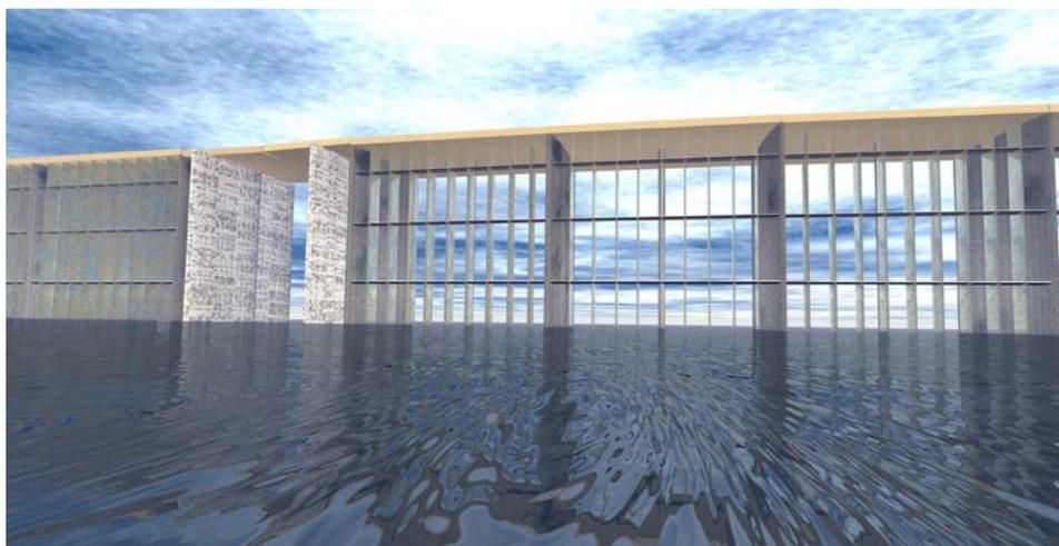
**Figure 9. The Eco-Barrier: Open, Ready for Business.** One surge gate is shown in the open position. There could be several such gates, to facilitate the passage of shipping. The height of the Eco-Barrier may be sufficient to pass shipping underneath; else drawbridges will be needed over the surge gates.
