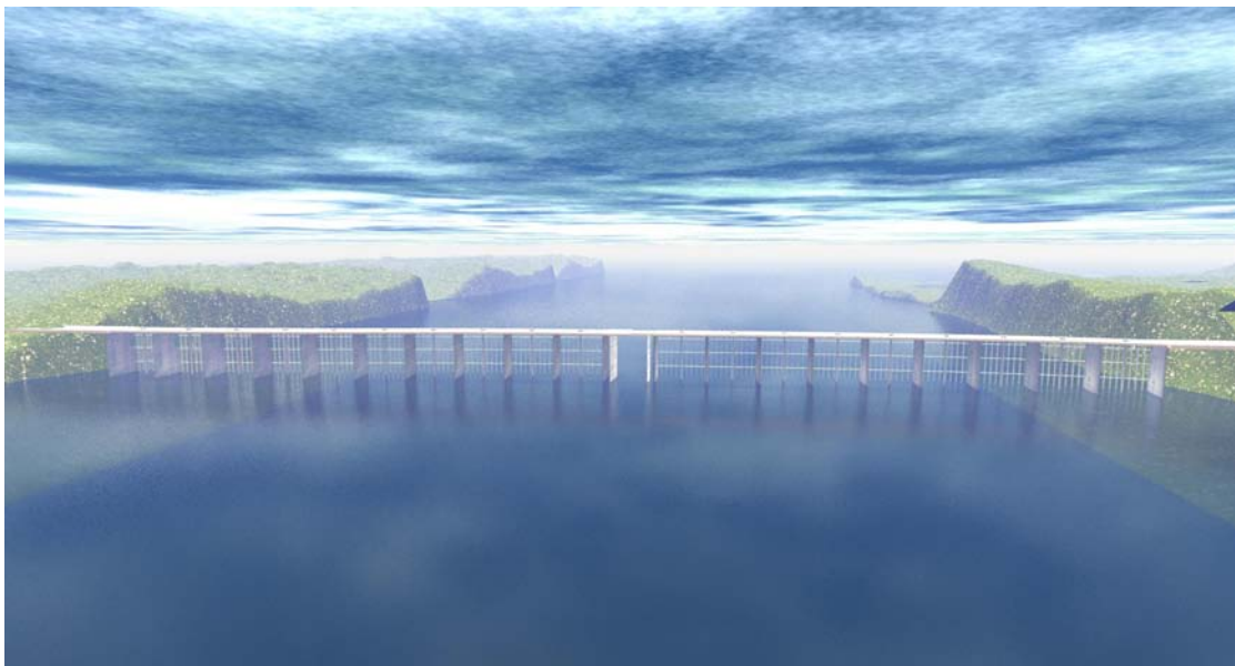
Figure 3. Severn Estuary Eco-Barrier Concept Many bays are connected together to form an Eco-Barrier across the opening, and between cliffs on opposing banks. Each bay is fitted with shutters, shown open. In addition there is an open lock (surge gate), to facilitate marine traffic. The whole offers little or no resistance to the flow of Estuary waters... Surge gates and shutters would be closed only to block Tidal Surge. Underwater turbines may be operating, but are not evident...The upper deck, in this artist's impression, is bare...but need not be in practice.
